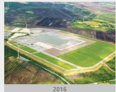
At the outset, a rehabilitation area was created by forming a tailings beach – a cap across the tailings management facility. This was followed by placement of a geotextile layer, which was covered with a rock cap. A growth medium of soil was placed across the completed rock cap.
